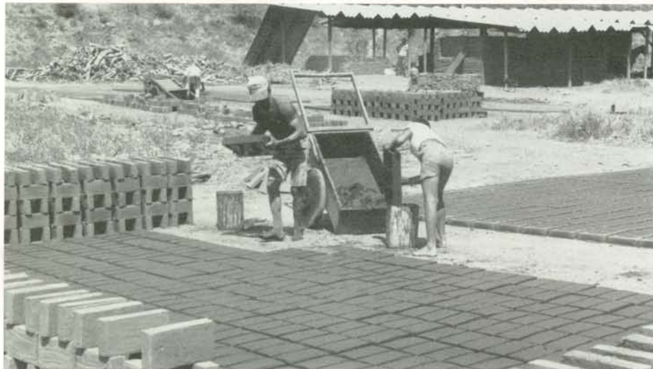
Brick making for TECHO-aided new housing construction.
