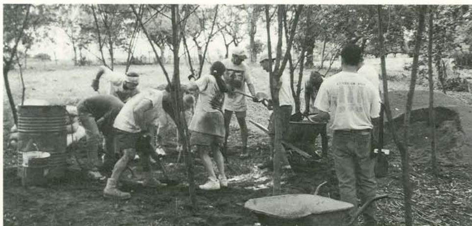
Villanova volunteers mixing cement for new classroom foundations at CENFAMA
